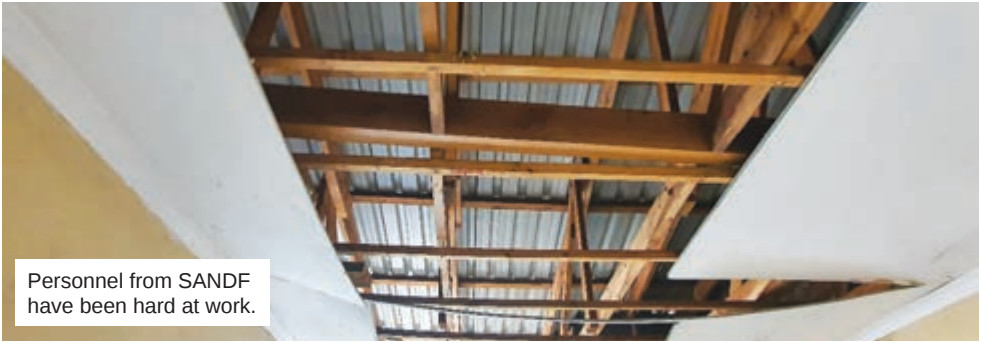
The renovations are still ongoing.
